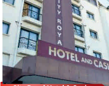
City Royal Hotel & Casino VRF Klima Sistemleri
